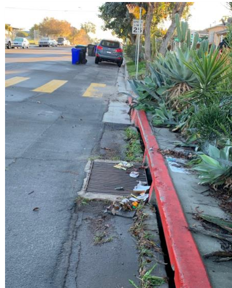
Accumulations of trash on a storm drain on an urban street in San Diego, where stormwater is untreated and conveys debris into receiving waters. 10 January 2020. Photo: T.S. Talley.
