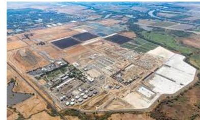
Regional San's wastewater treatment plant upgrade aims to produce cleaner water for discharge to the Sacramento River (Photo: Regional San).
