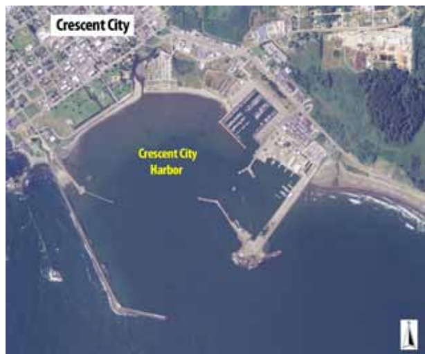
Figure 1. California map locating Crescent City and aerial view of Crescent City Harbor.
