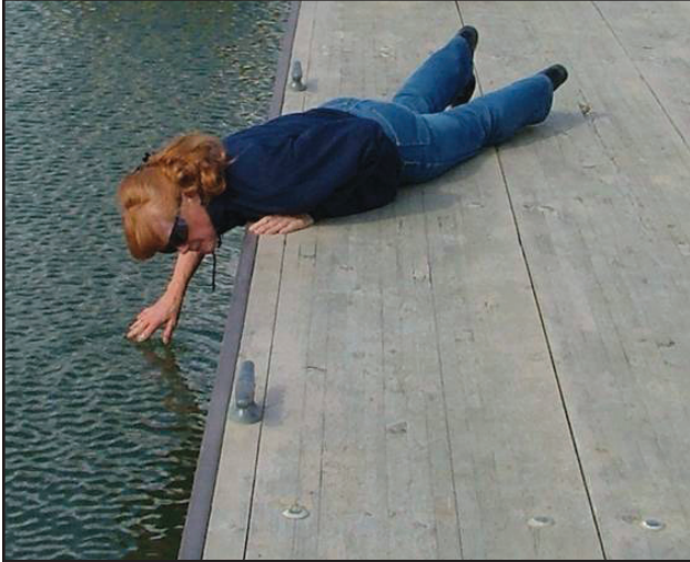
Figure 12. Visual inspection of dock undersurface. Photograph courtesy of California Department of Water Resources.
