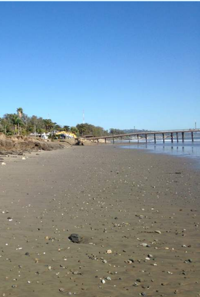
Figure B1. Extreme beach erosion at Goleta County Beach during the 2015–2016 El Niño (Photo: D. Hoover, USGS).
